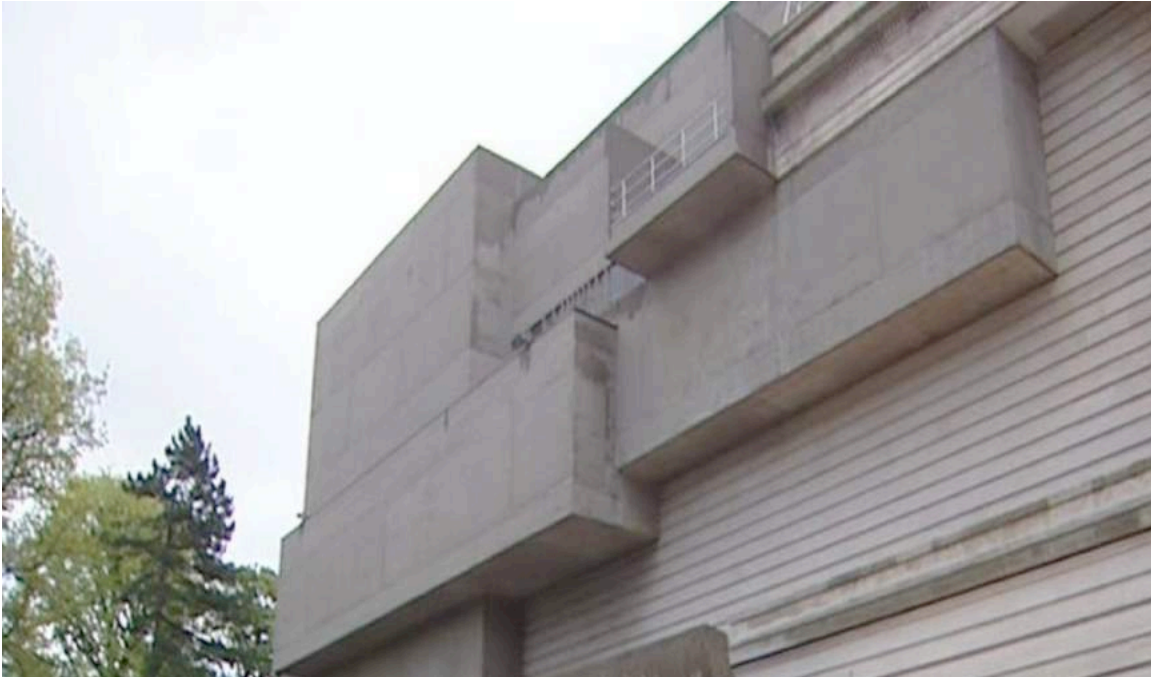
The concrete blocks of the Pym extension
