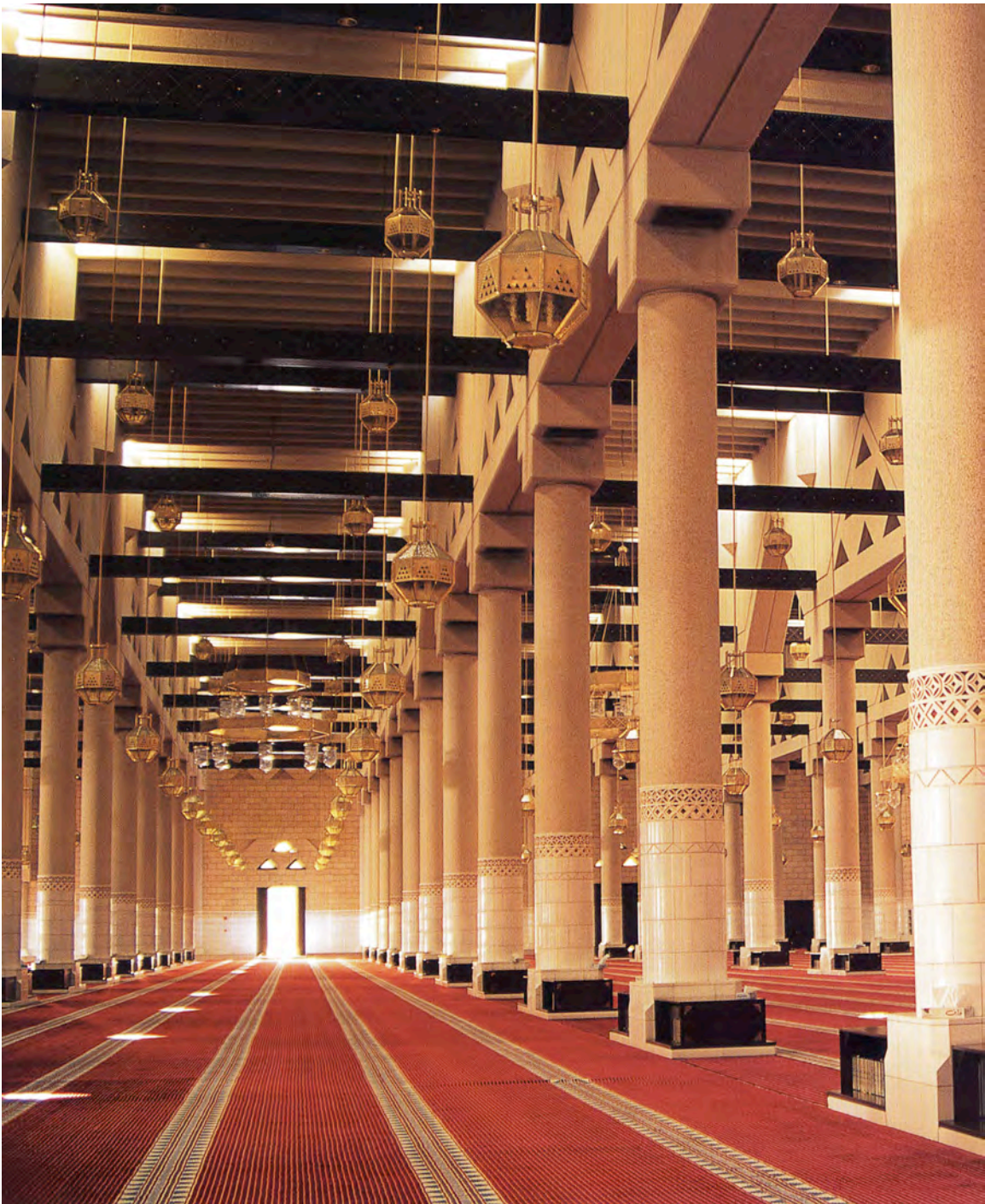
Page 74: Great Mosque, Riyadh, Saudi Arabia. The hypostyle, or many-columned hall, has a long history in Islamic architecture, even though the technology now exists to enable a more open structure to be used.
