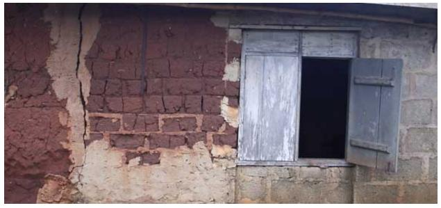
Close-up of a wall section, graphically depicting Iwesi builtform in historical progression: to the left, cob construction typifies the earliest building tradition; in the middle, repair-work was effected in earth bricks, sand-cement- earth-bonded; to the right, is the latest repair job, featuring sand-cement blocks. Jump to Images of Iwesi
