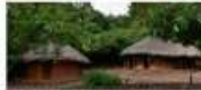
Earthen houses built on a mound with a round verandah protecting the walls from the rain. (Credit: Omo Zone in SWPP). ©: Enriquer Sevilano
