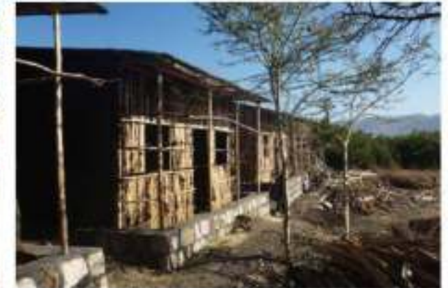
New chikka houses under construction in Amhara region. CC- Canned Muffins
