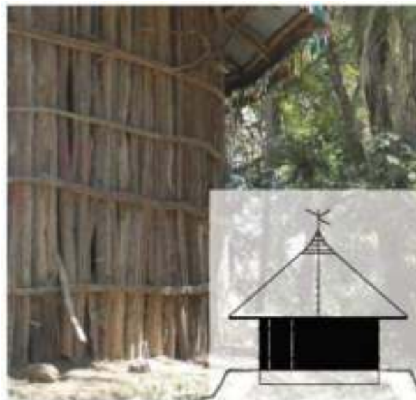
This church (Bura, Amhara) lies on an earthen mound to protect against floods. There is a corridor between the interior earth wall and the wooden exterior wall. These two elements prevent from the effects of black cotton soils expansion if the platform is built with inert earth, and so cracking of walls is avoided. © L. Davis
