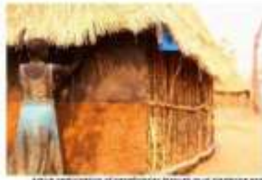
Active participation of beneficiaries through mud plastering and thatching. © IOM/UNHCR/ARRA
