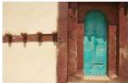
Church of Kibbe Afba with monkey head technique in the walls. Yeha, Tigrai. cc-A. Dery
