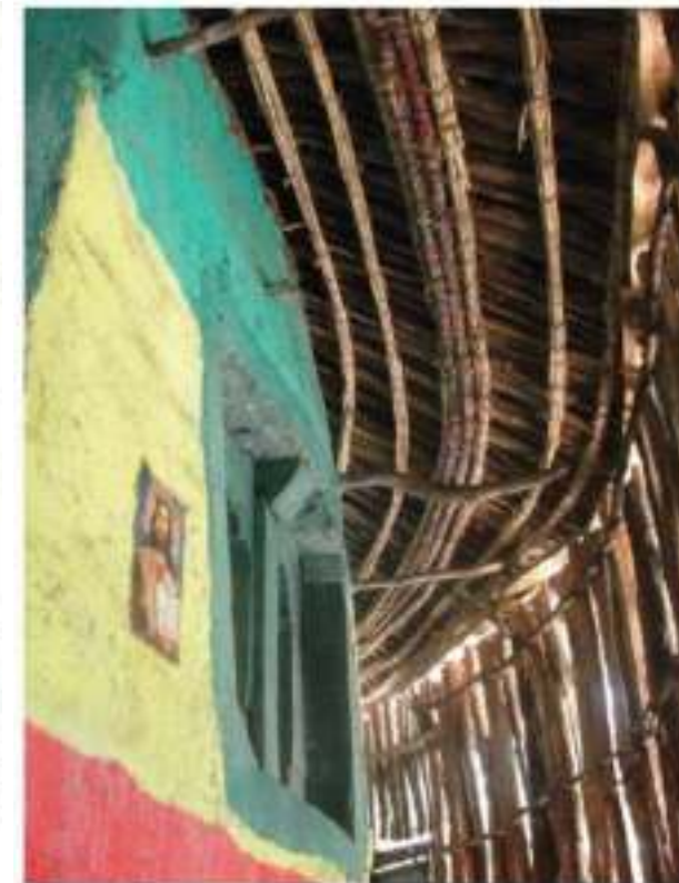
Church in Bura (Amhara) with an inner block built with chikka protected by a roofing with a very large overhang that creates a verandah surrounding the entire building. An eucalyptus screen helps protect the chikka mortar and the foundations of the inner block from black cotton soils cracking. © L. Davis
