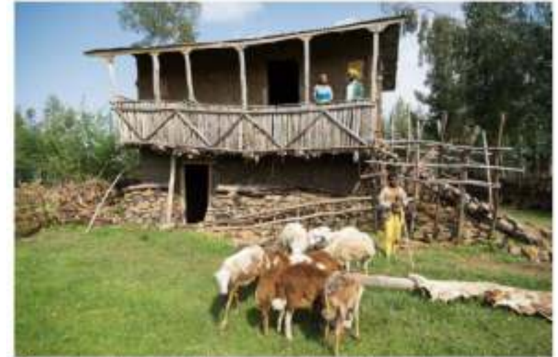
Two story house with stone plinth, chikka walls and balcony in Gobgob village, Amhara region. CC- Kelley Lynch USAID
