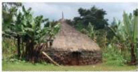
Sidama people house built with a bamboo structure and a vegetal covering for walls and roof. cc-Mauris V.
