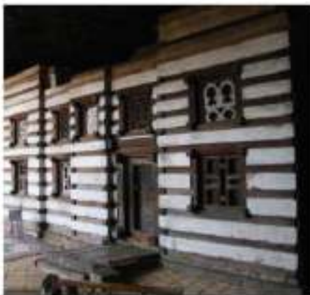
Church of Yemrehanna Kristos with horizontal timber bands or «monkey heads» near Lalibela in Amhara. CC-Travel Aficionado
