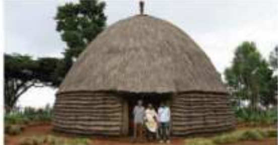
Welayta people house built with a bamboo structure and a vegetal covering. © Todd McQueen
