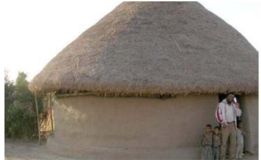
Ventilation is made possible thanks to the absence of plaster in the upper part of the walls in the Alaba houses (SNNPR). © Lorenzo Fontana
