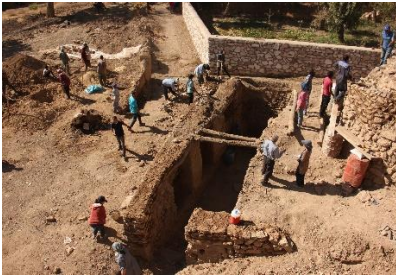
Figure 9) The chamber after excavation ©Sonia Beigi
