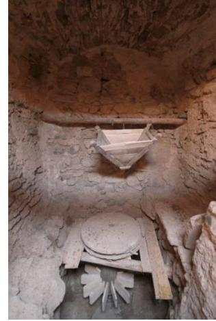
Figure 6) Final picture of reassembled the wheel ©Sonia Beigi
