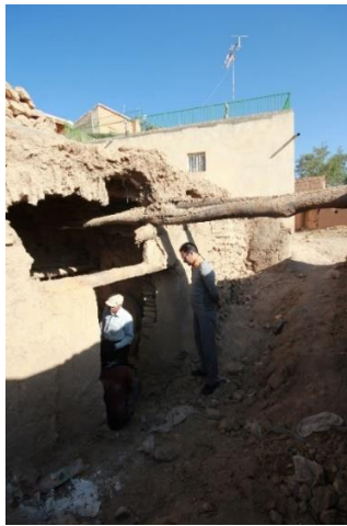
Figure 7) The chamber after excavation ©Sonia Beigi
