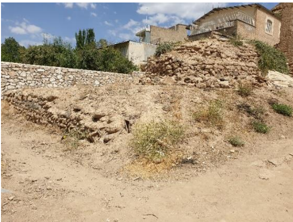
Figure 17) initial condition of the abandoned watermill ©Sonia Beigi
