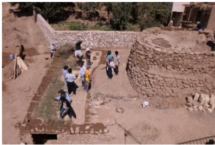
Figure 12) Chamber ceiling reconstructing procedure ©Sonia Beigi
