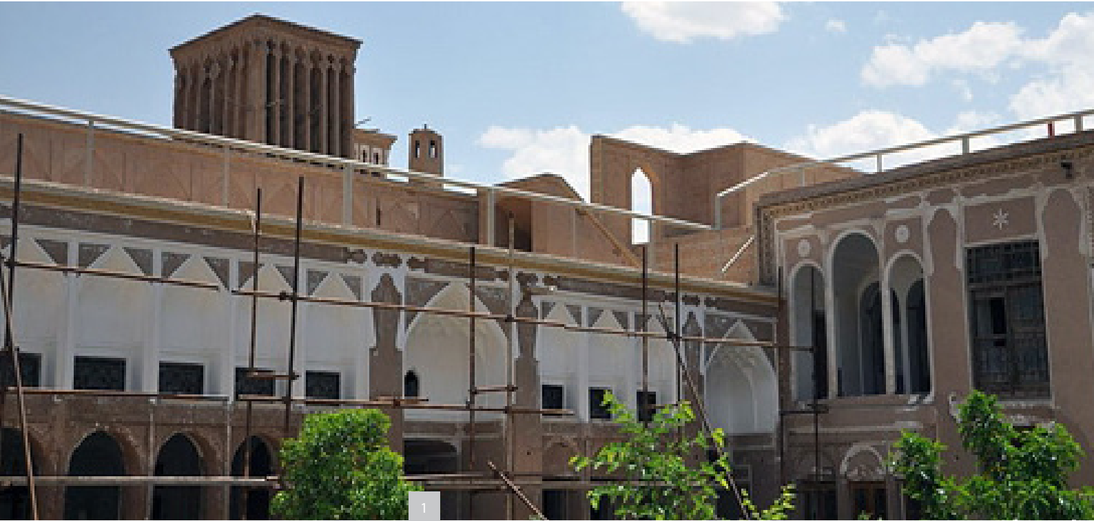
Images 1&2- Iqbal factory during renovation
