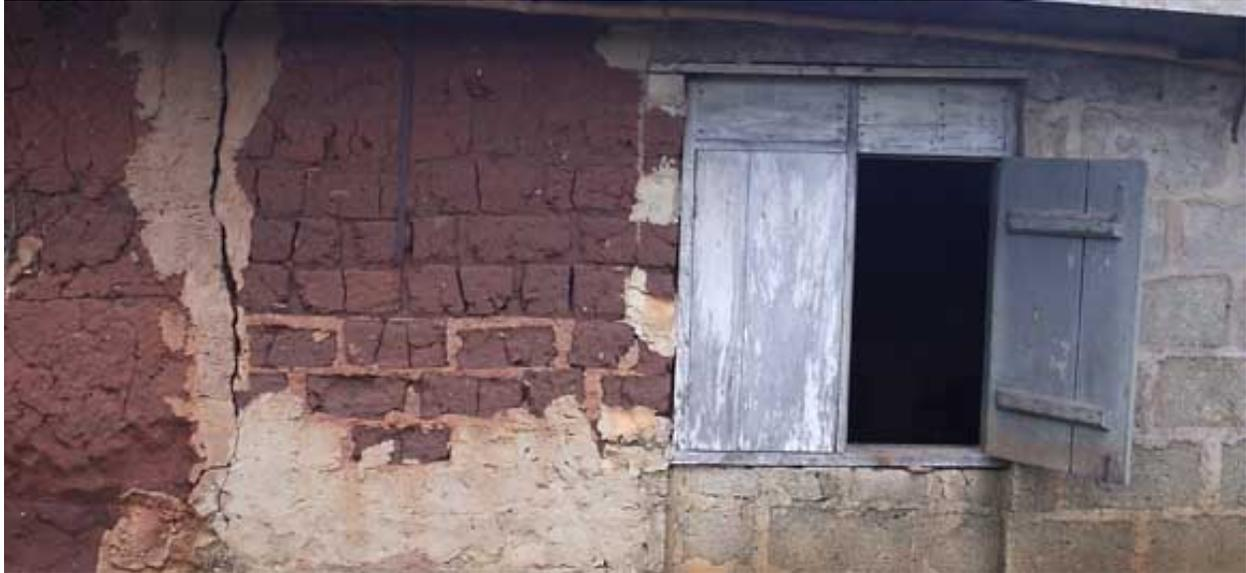
*Close-up of a wall section, graphically depicting Iwesi builtform in historical progression: to the left, cob construction typifies the earliest building tradition; in the middle, repair-work was effected in earth bricks, sand-cement- earth-bonded; to the right, is the latest repair job, featuring sand-cement blocks. Jump to [Images of Iwesi](#)*
